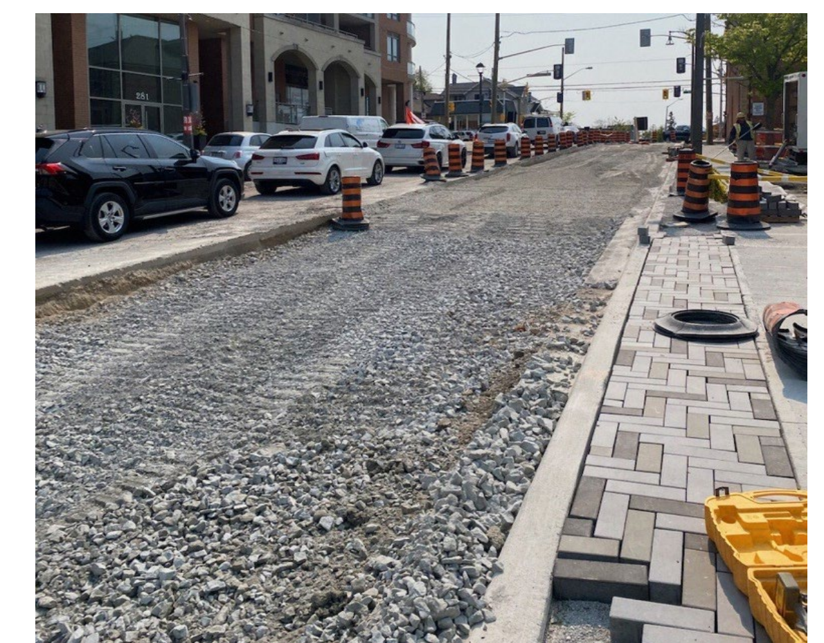
Typical paver stone interlock installation
